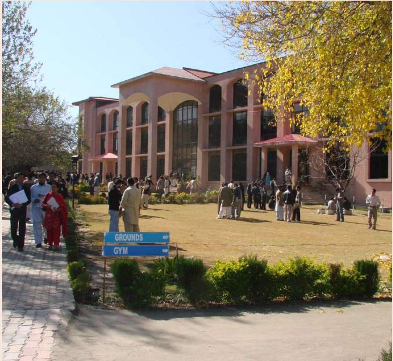
Engineering Block at CIIT Abbottabad
